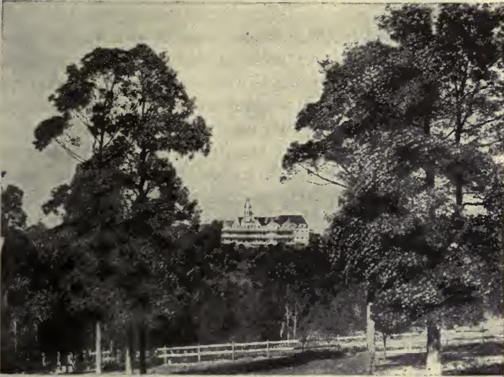
A sanitarium in the forest
